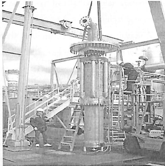
Fig-15 LNG Send out Pump
