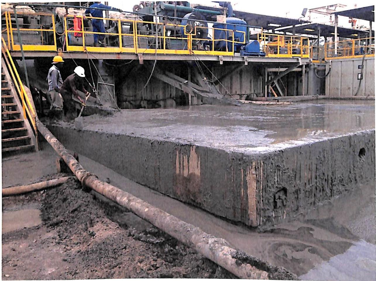
*Figure 1.1: Waste pit overflowing*
