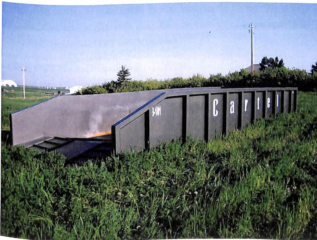
*Figure 4.3: Example of a Three Sided Shale Bin*
