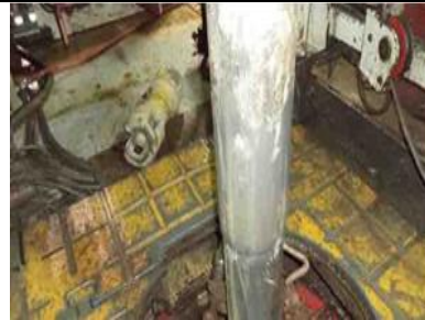
Figure 24: Clamp Fell on rig floor
