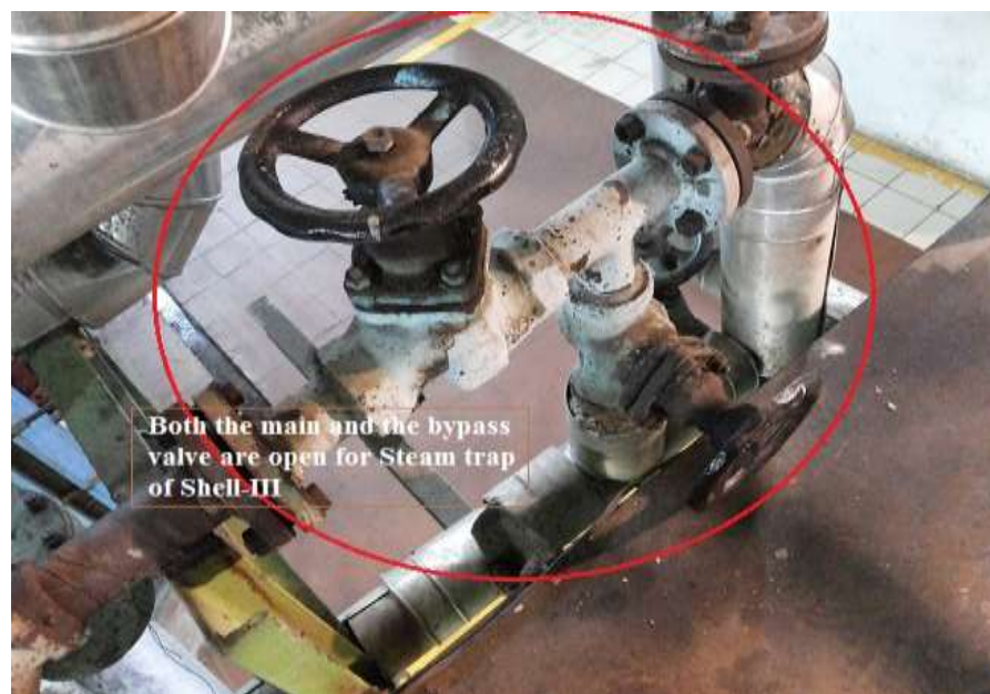
Fig 4.15(c): Opening of both main and bypass valve of steam trap of Shell-III
