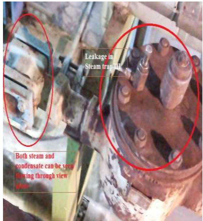
Fig 4.15 (b): Steam trap of Shell-III
