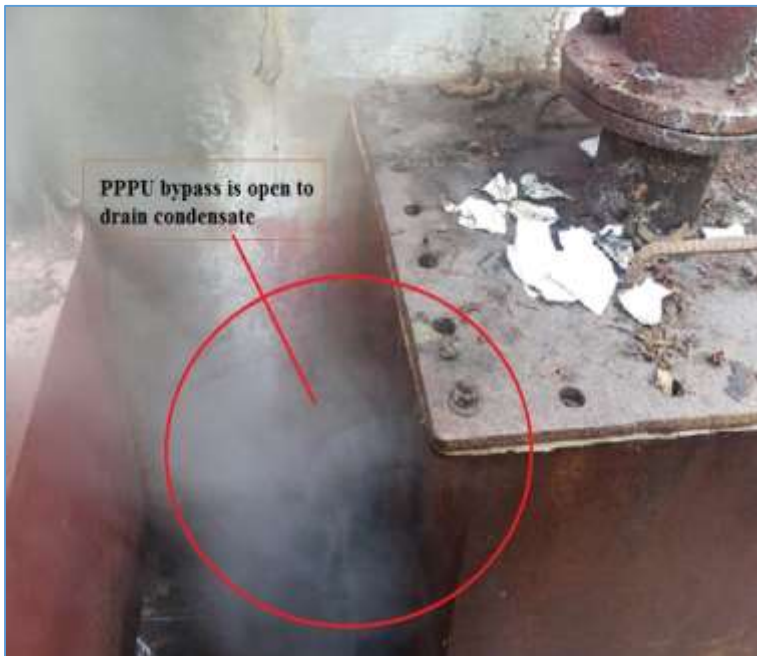
Fig 4.15 (d): Bypass of PPPU opened
