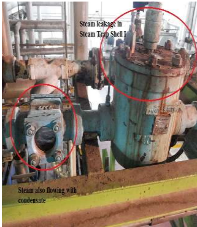
Fig 4.15(a): Steam trap of Shell-I
