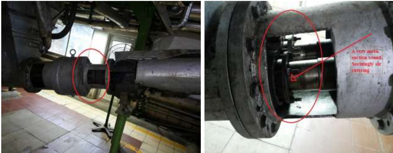
Figure 4.18 : Screw Discharge at the bottom of cone section of WFE
