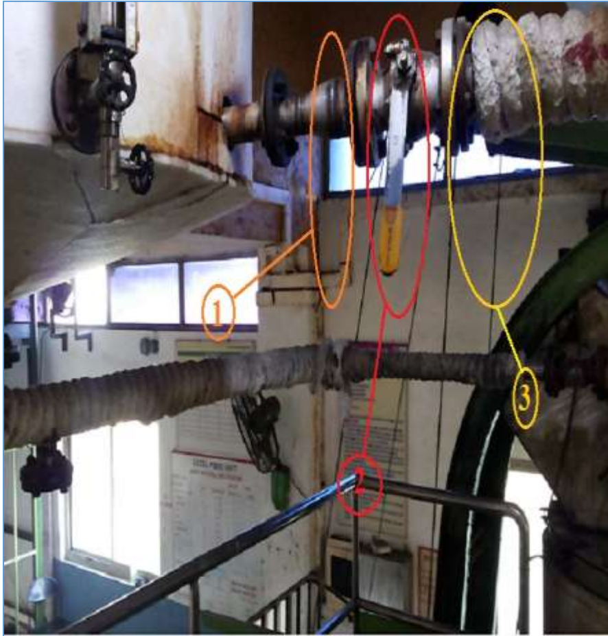
Figure 4.9: Valve restructure point of 10TPD pulper overhead tank
