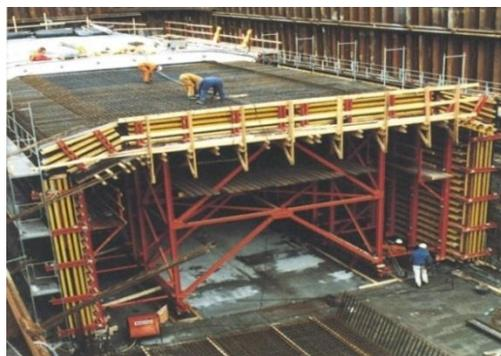
**Figure 1.2: cut and cover method**
