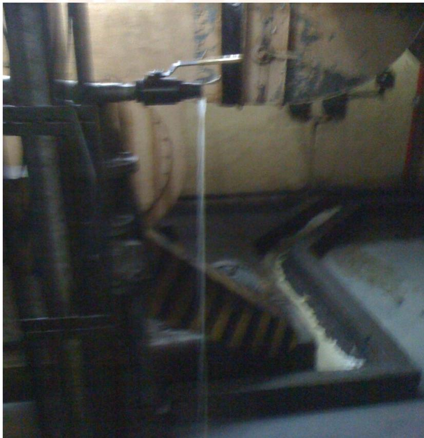
**Fig 5: Leakage at Grinding Basement**
