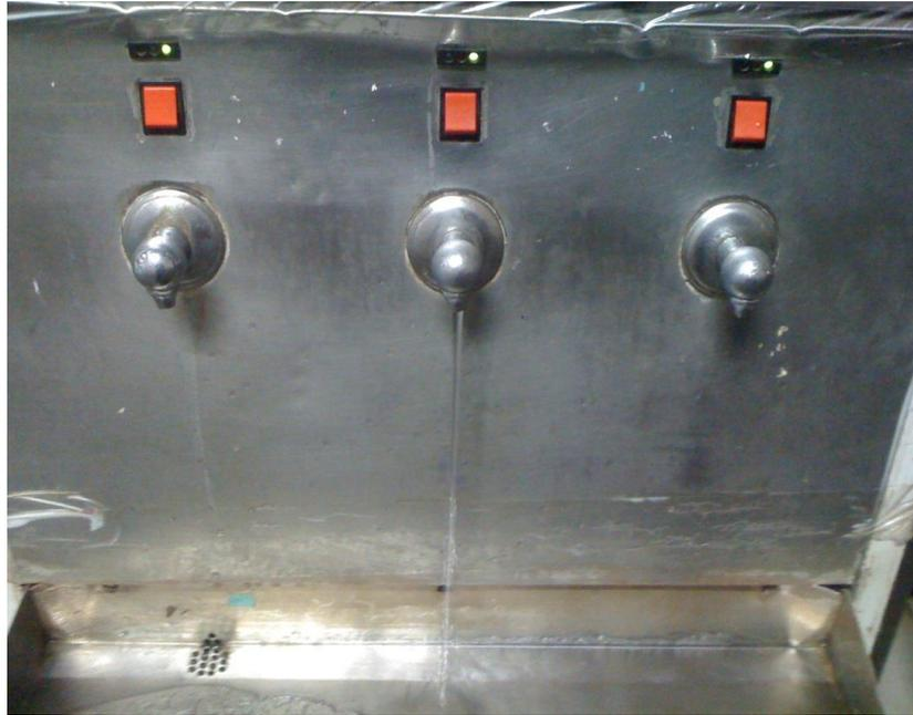
**Fig 4: Leakage at Water Cooler**
